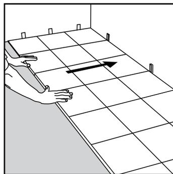
**[9]** The distance to the walls can be adjusted when three rows are completed. Remember to place the flooring a minimum of 1/4" from all walls or other vertical obstructions such as cabinets, pipes, or columns.
