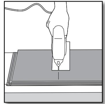
**[5]** Place the plank face down on the work surface and cut to size with a power saw. If you are using a hand saw, use a fine-toothed blade, and cut the planks face up.
