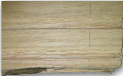
Bottom of Board Defect
